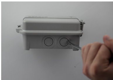
Fig. 1: Punch cable hole
